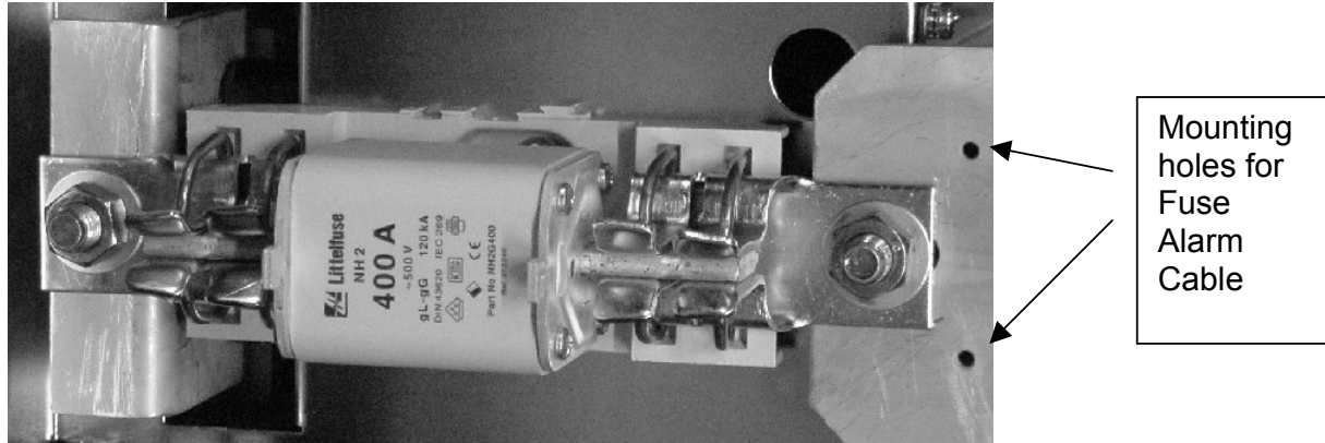
Figure 3.7-6 NH2 Fuse Connections
