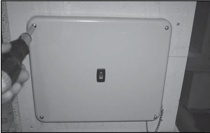
Figure 6.3 Remove Control Cover
