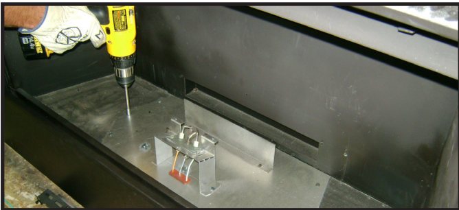
Figure 11.2. Remove Valve Plate Screws
